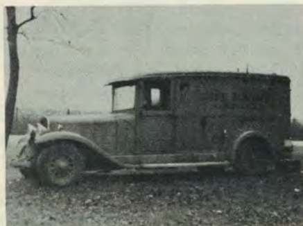
District Aux. Comm. Truck, equipped with 2 Transmitters and Receivers, 1 battery operated, 1 AC power, 50 watts output.
