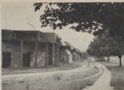
Rear of Fort Mott—dismantled gun pits.
