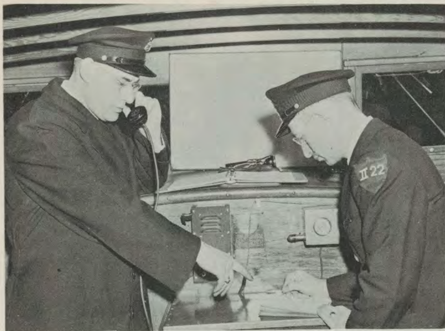
Communication with Headquarters via Ship-to-Shore Radio
