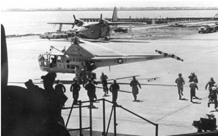
Below: Air Station Brooklyn Source: U.S. Coast Guard Historian's Office
